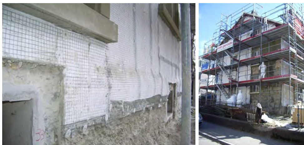
Fig. 24 Retrofit wall insulation with Spaceloft blankets. Wall and window sill detail ( left ) and house side-on view ( right )
