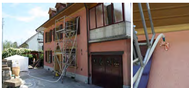
Fig. 20 Cavity wall insulation with aerogel granulate in Biel, Switzerland. View of the renovation site (left) and zoom on the injection hole (right)
